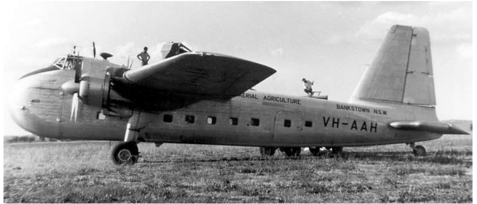
Bristol 170 Freighter VH-AAH having its removable internal hopper loaded with fertiliser at Cootamundra in 1958. (Photograph by Ben Dannecker)
